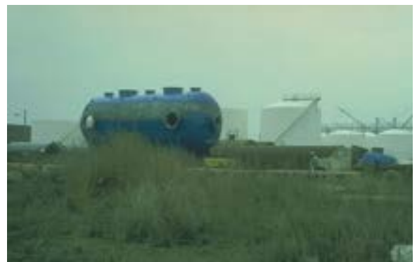
Above ground storage tanks
